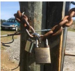
One of the responses to our questionnaire was that the gate locking chain was confusing and "would defeat Houdini". This was made evident when someone inadvertently used the Ranger's lock and locked us out of the field. The chain system has now been simplified. There are now only two locks. The silver one is the Rangers and the brass one is TMAC. The chain has been shortened such that it is unlikely that the chain can be connected without both padlocks in series.
